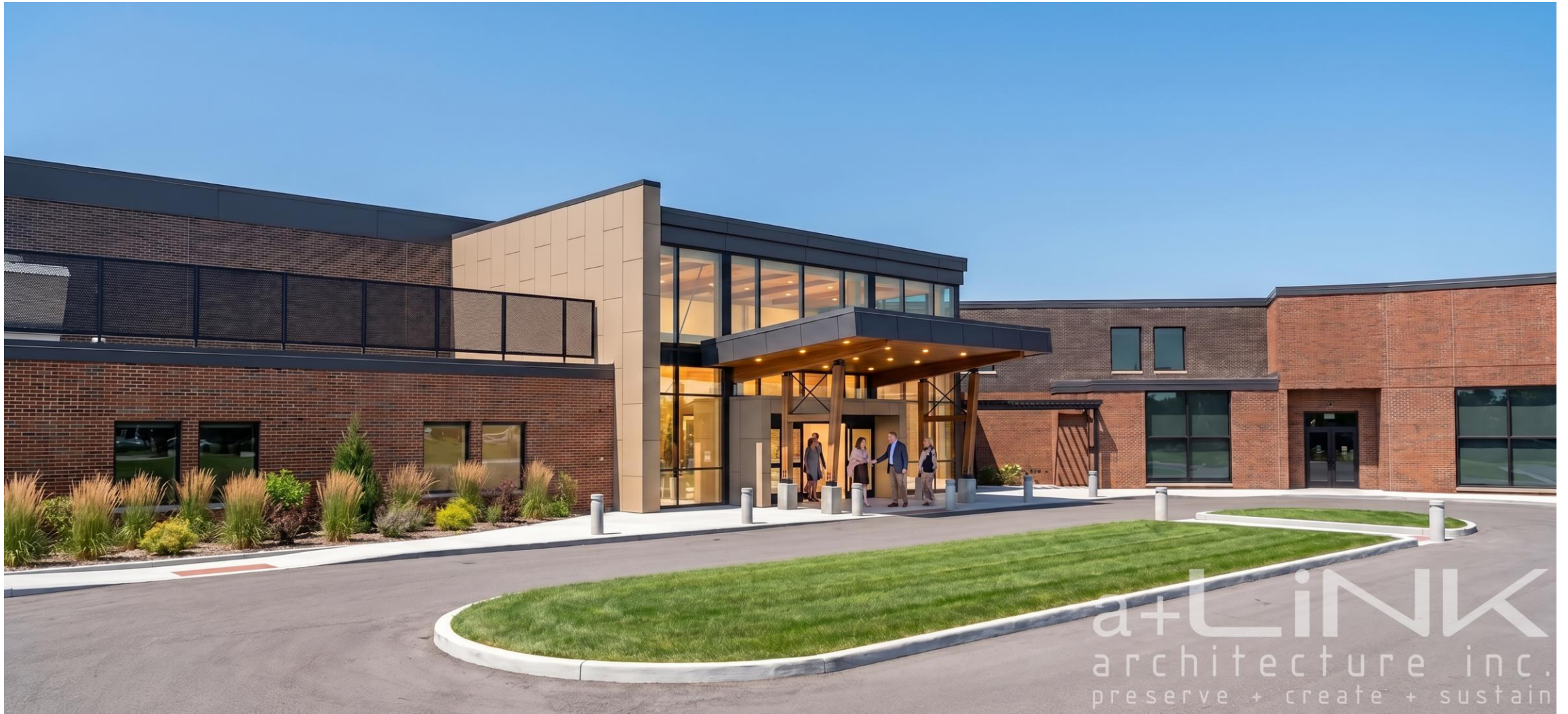
New Front Entrance – View from left side of the parking lot as you walk into the building
